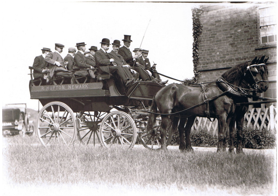
A tour of the works – at Beacon Hill
