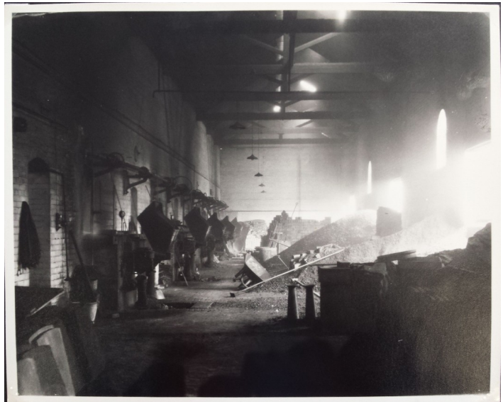
Furnaces at Beacon Hill (Photo Courtesy of Saint Gobain)
