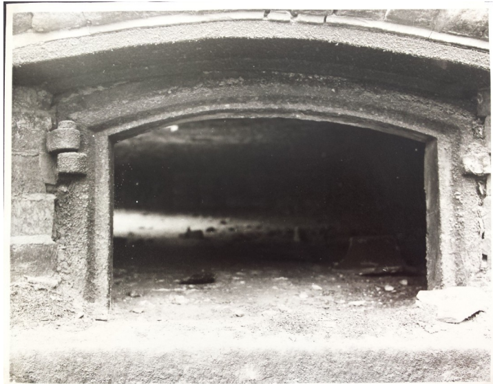
The doorway to an old Keenes Oven (Photo Courtesy of Saint Gobain)
