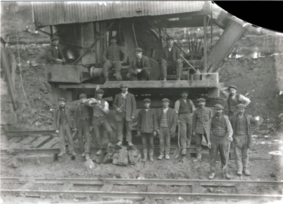
The Ruston Excavator at Hawton
